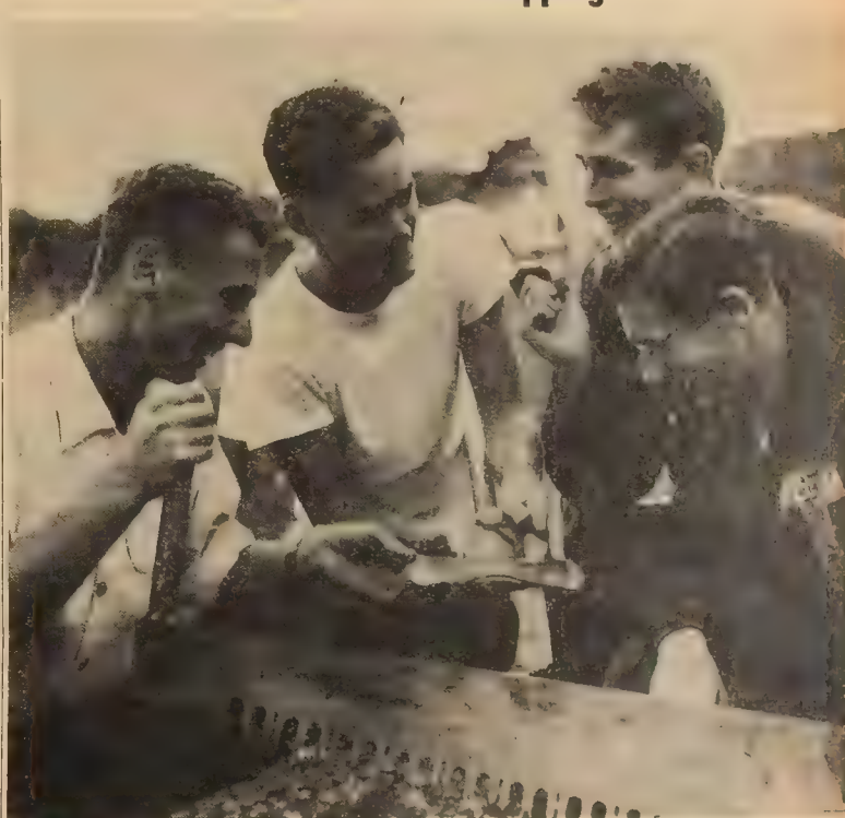
Gerry Helleiner, Rich Newman and Terry Byram cut trees in the orchard of the Caledon Hills Farm. Victoria and Trinity freshmen planted trees, mended the roof and replaced windows as part of their "constructive" initiation. — VSP Ed Staworzynski
